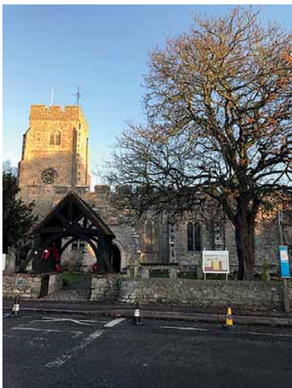
The parish Church of Eastchurch, at the heart of the village.
