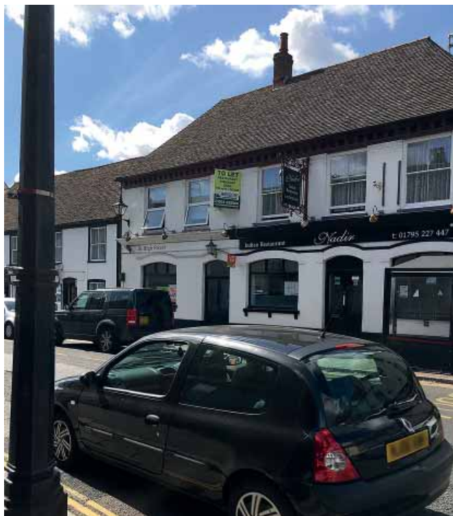
89-91 High Street, Milton Regis (a grade II listed building). Unauthorised finow replacement work is being tackled by the Council
